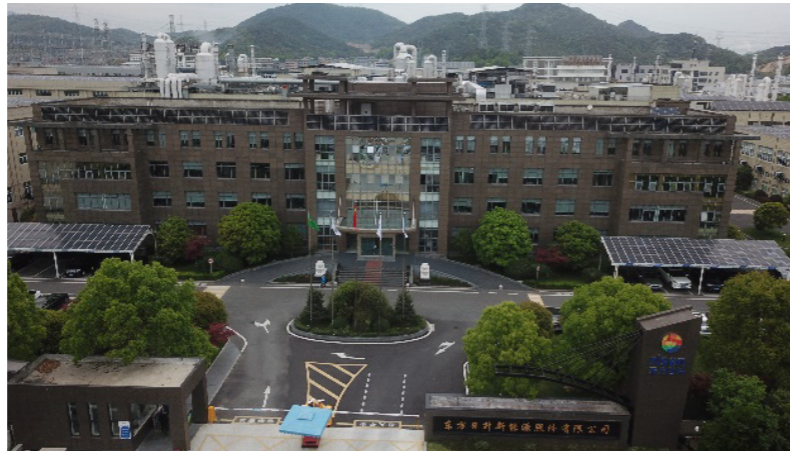
Installation Site: Group headquarters Size of the System 1.5MW
