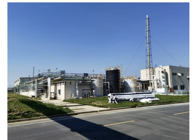
Sewage Treatment Station
